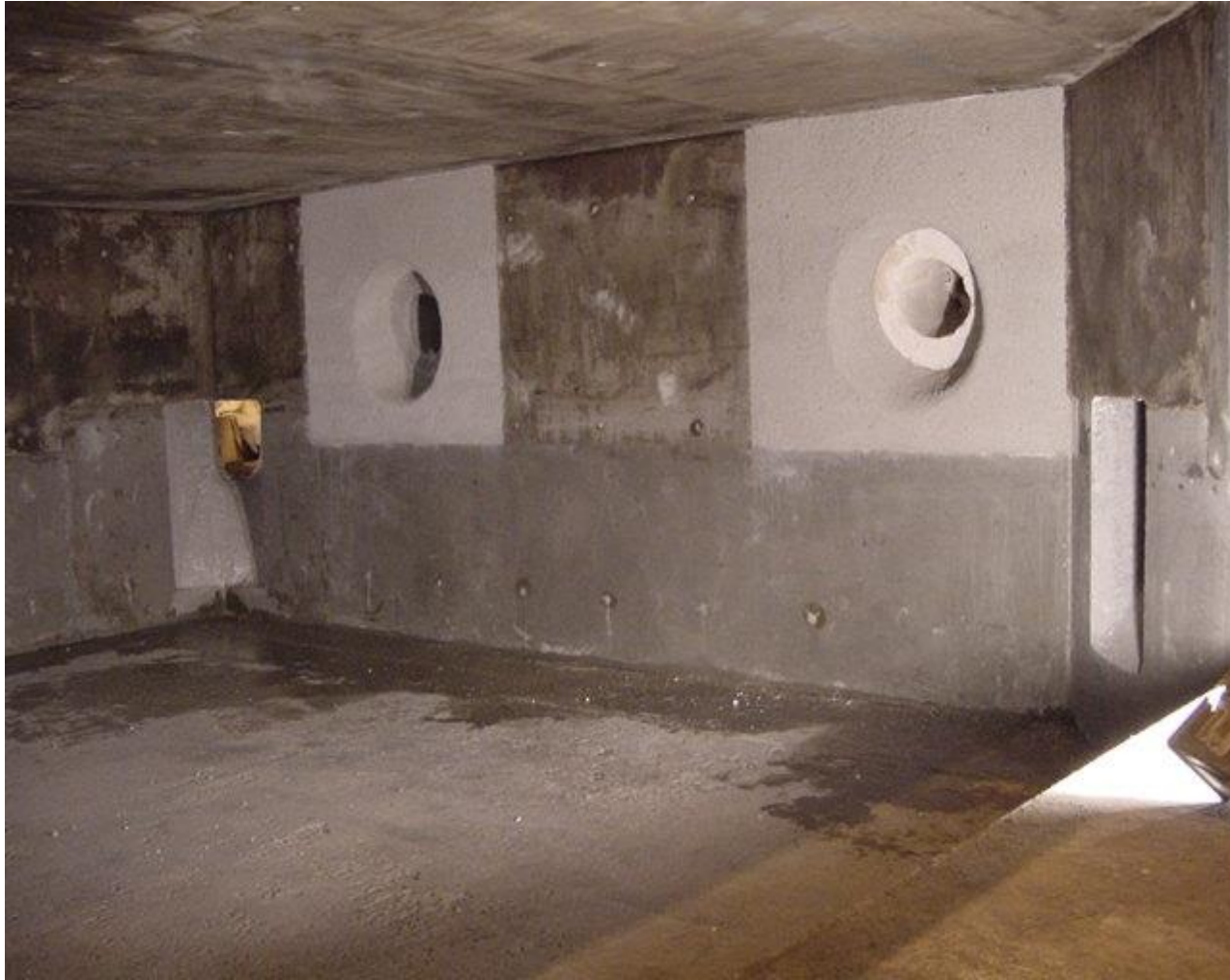
40T Holding Furnace - UK
