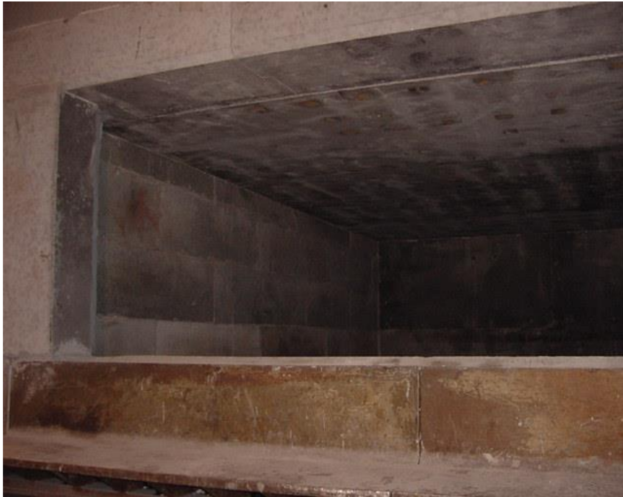
65T Side well Melting Furnace - UK
