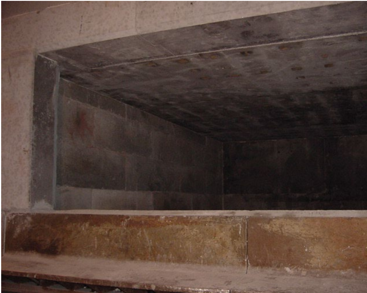
65T Side well Melting Furnace - UK
