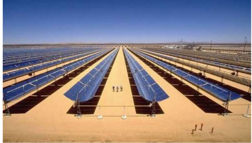
Figura 22.14 – Colector Solar Concentrador
